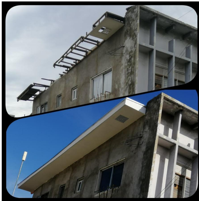
Bible Study Center (BSC) building final repair
